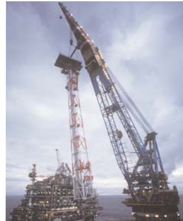
Micoperi 7000, Flare installation, Bruce Field, North Sea, Off UK 1991
