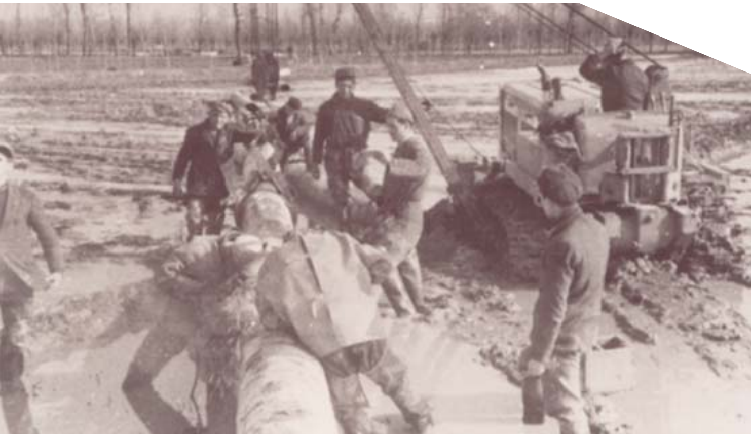
Line up and Welding, Snam Gas Line System, Po Valley, Italy, 1953
