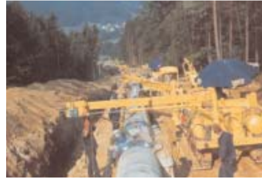
Line up by cable car, 36" Gas Line from Czech border to Italy, Austria, 1972
