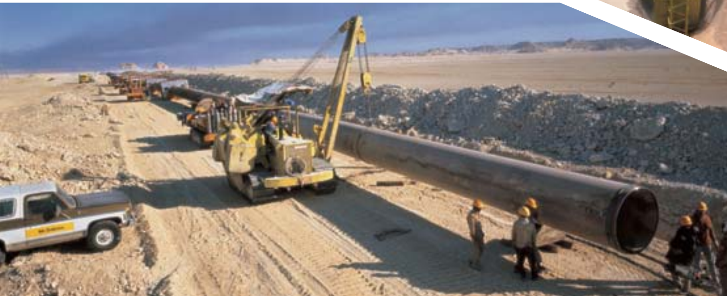
Line up and welding, 56 Khurais to Yanbu Oil Line, Saudi Arabia, 1987
