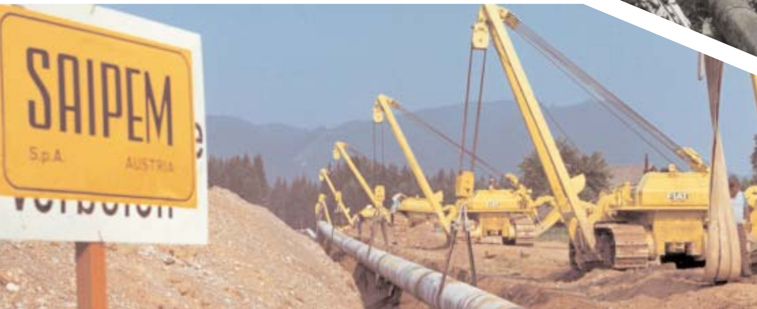
Laying and Tie in, 36" Gas Line from Czech border to Italy, Austria, 1972
