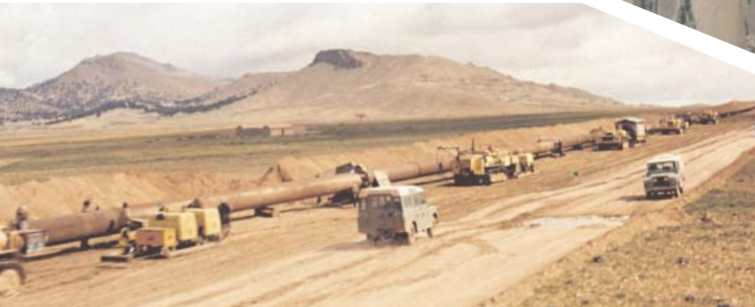
Welding, 48 Transmed Gas Line, Tunisia, 1979
