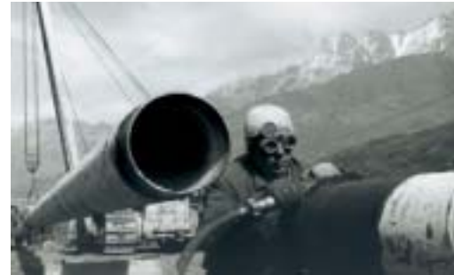
Line ready for the lowering in the ditch, 26 Oil Line Genoa - Ingolstadt, Forest near Memmingen, Germany , 1963
