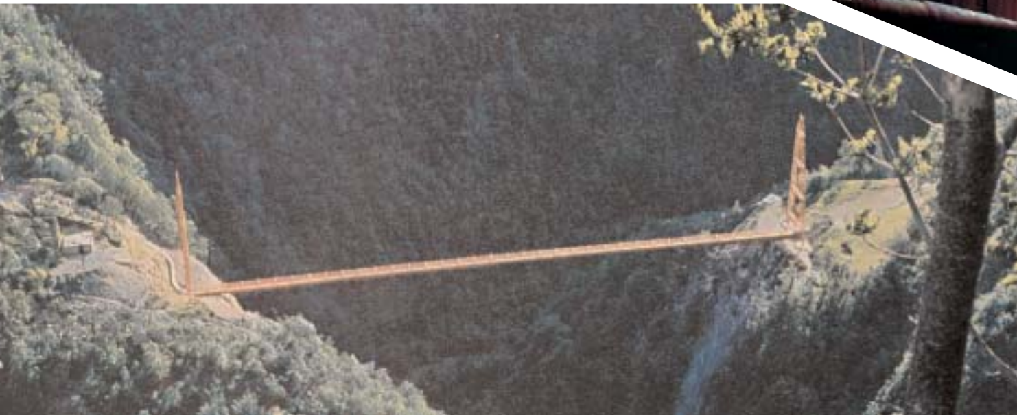
Bridging a narrow valley, 26 Oil Line Genoa - Ingolstadt, Varrone river, Italy, 1961
