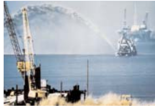
Castoro 10 and Castoro Sei, Trenching and Laying, 20 & 30 Sealines Dong Project, North Sea, Off Denmark, 1983
