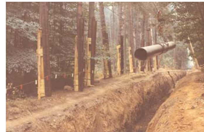
Stringing by cable car, 36" Gas Line from The Netherlands to Italy, Germany, 1972
