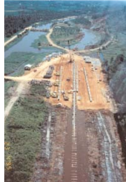
Launching Yard, 36 PGU III Gas line, Malaysia, 1996
