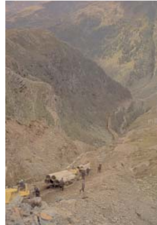
Pipe stringing, 26 Oil Line Genoa - Ingolstadt, Alps Crossing, Italy, 1962
