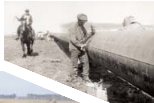
Weld Cleaning, 30 Gas Line Santa Cruz -Buenos Aires, Argentina, 1962
