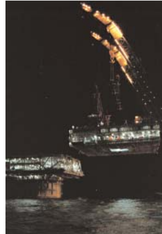
Saipem 7000, upper module installation in DP mode, Diana- Hoover Project, Gulf of Mexico, Off USA, 1999
