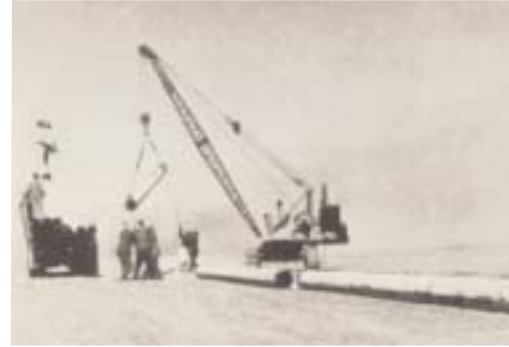
Coating and laying, 16 Oil Line Gahuati - Siliguri, India, 1960
