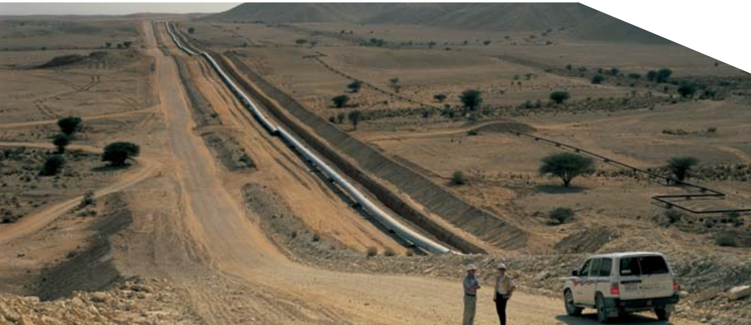
Pipeline ready for installation in the ditch, 56 Hawiyah Gasline, Saudi Arabia, 1999
