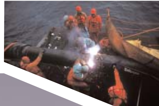
Castoro II, above Water tie-in, 22 Gasline across Gibraltar Straits, Off Spain, 1995
