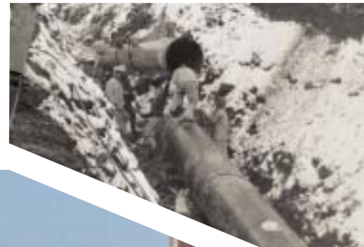
Line up by cable car, 36" Gas Line from Czech border to Italy, Austria, 1972
