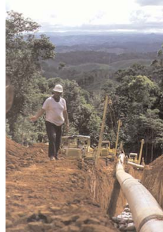
Laying, 30 Vasconia-Covenas Oil Line, Colombia,1995
