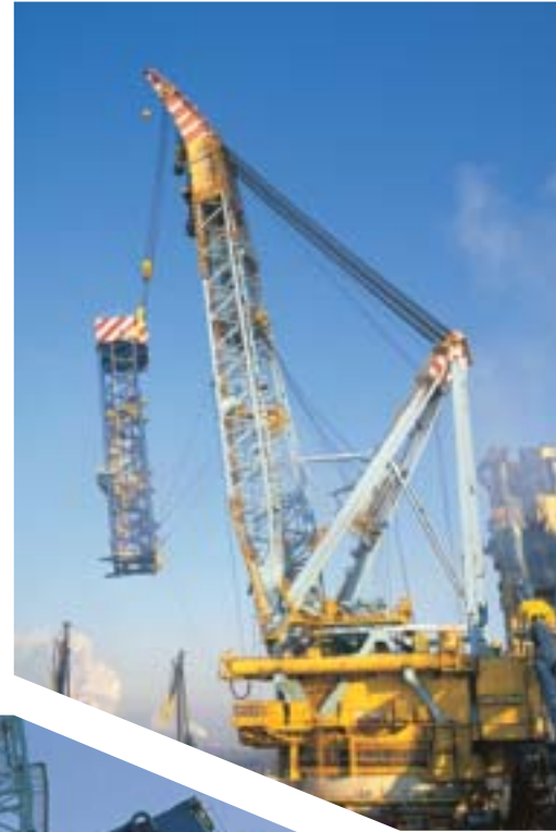
Saipem 7000, installation of the upper portion of the J-lay Tower, Rotterdam, The Netherlands, 1999
