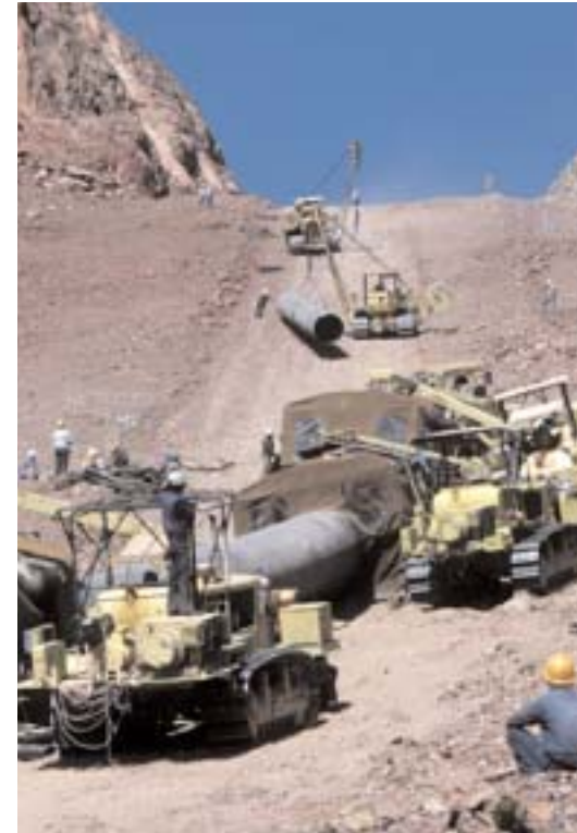
Line up and welding, 56 Khurais to Yanbu Oil Line, Saudi Arabia, 1987
