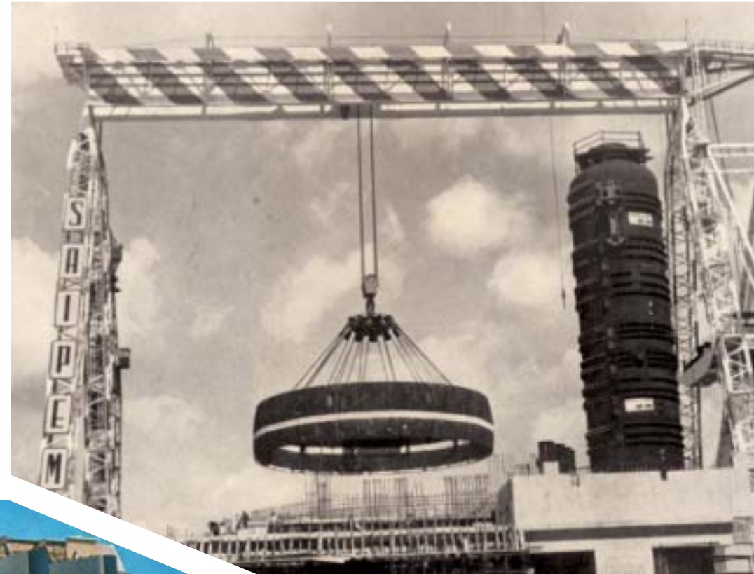
Installation of a ring of the reactor containment sphere, Nuclear power plant, Latina, Italy, 1960
