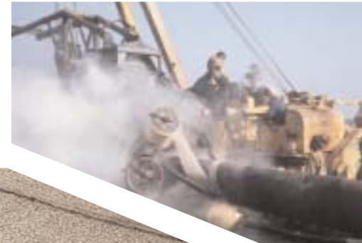
Coating and laying, 16 Oil Line Gahuati - Siliguri, India, 1960
