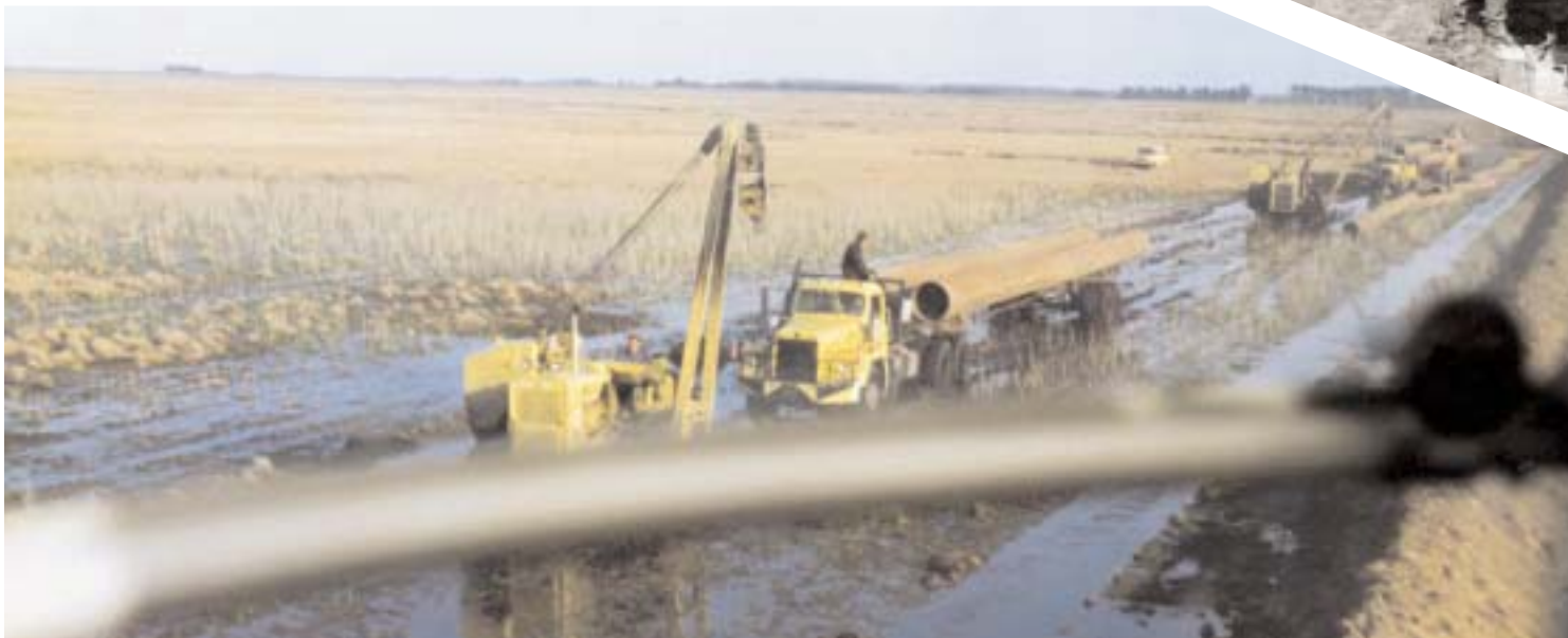
Stringing in flooded pampas, 30 Gas Line Santa Cruz - Buenos Aires, Argentina, 1962
