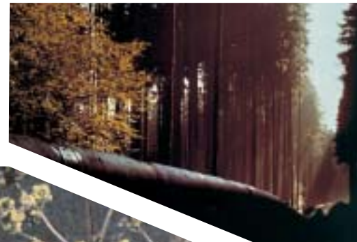
Line ready for the lowering in the ditch, 26 Oil Line Genoa - Ingolstadt, Forest near Memmingen, Germany , 1963
