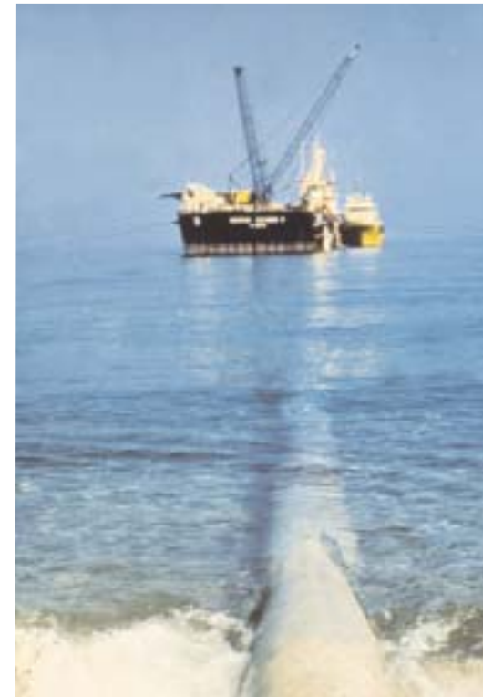
Castoro 5, Landfall, 10 Gas Sealine, Messina Straits, Italy, 1974
