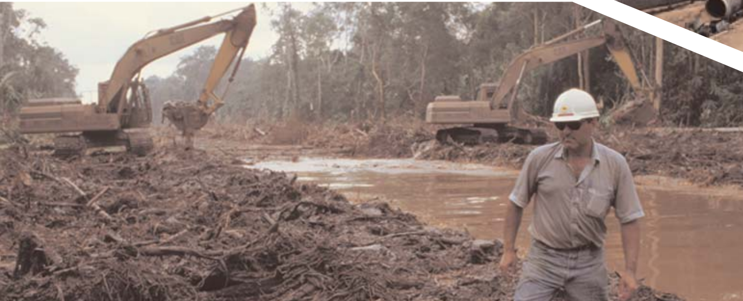
Trench Preparation, 36 PGU III Gas Line, Malaysia, 1996
