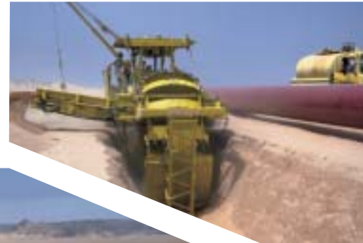
Ditching, 56 Khurais to Yanbu Oil Line, Saudi Arabia, 1987
