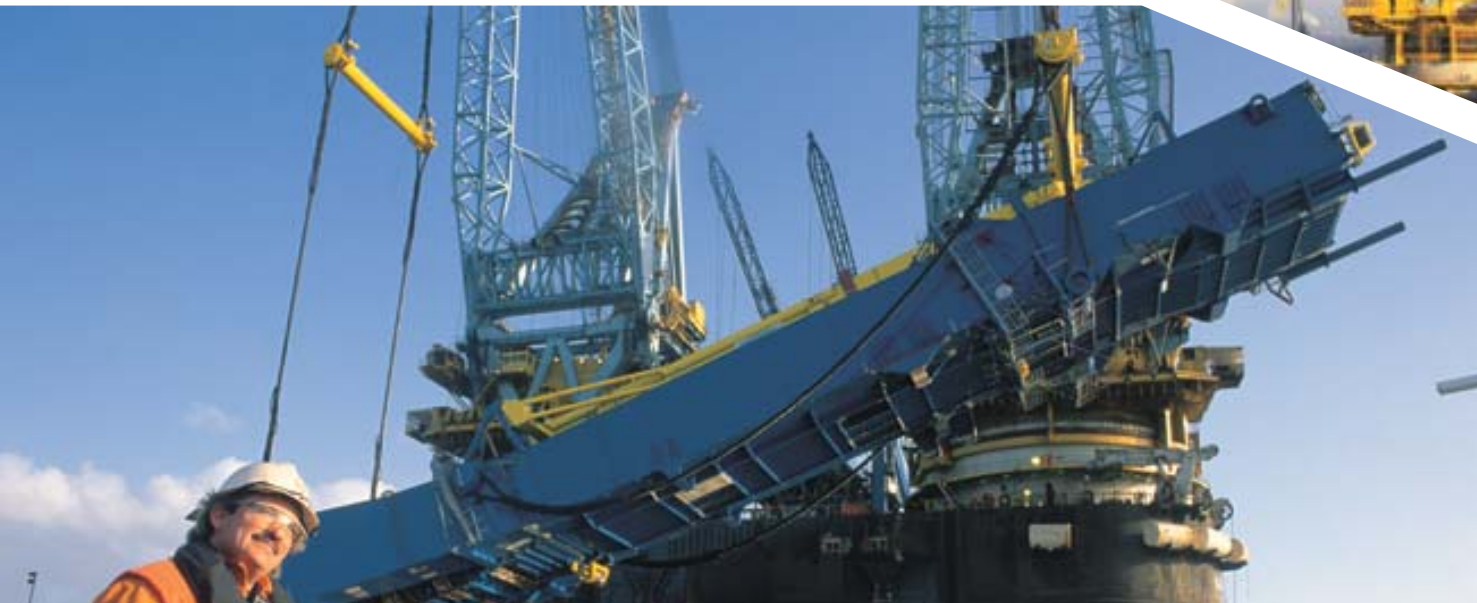
Saipem 7000, installation of the lower portion of the J-lay Tower, Rotterdam, The Netherlands, 1999
