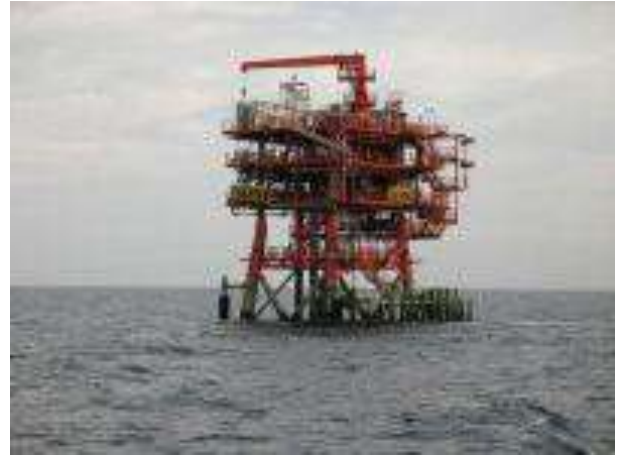
Calipso production platform
